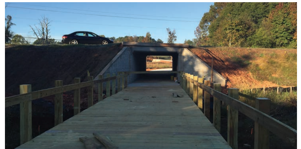
Multi-use trail through existing box culvert requires a 7'6" minimum vertical clearance.
