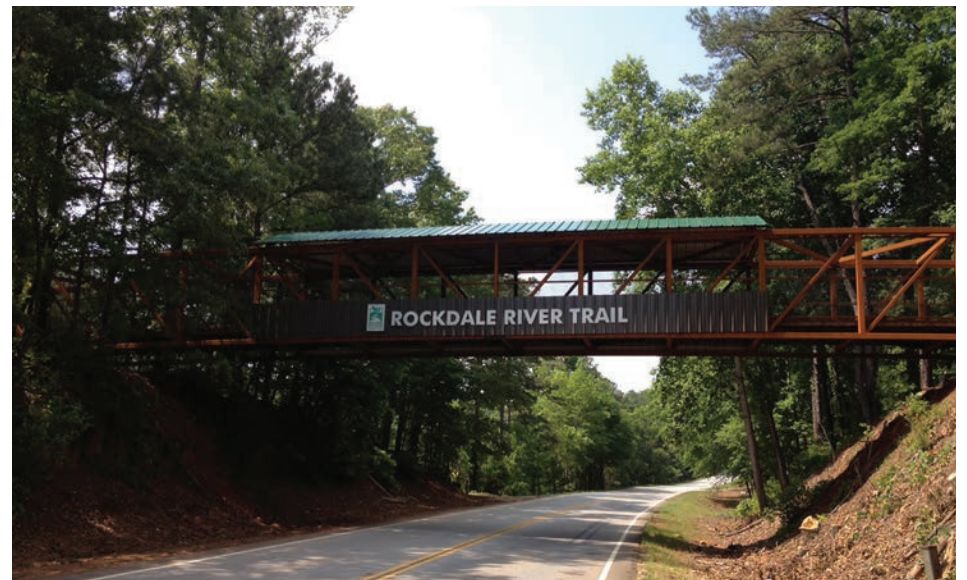
Prefabricated steel bridges allow trail to cross above existing roadways.
